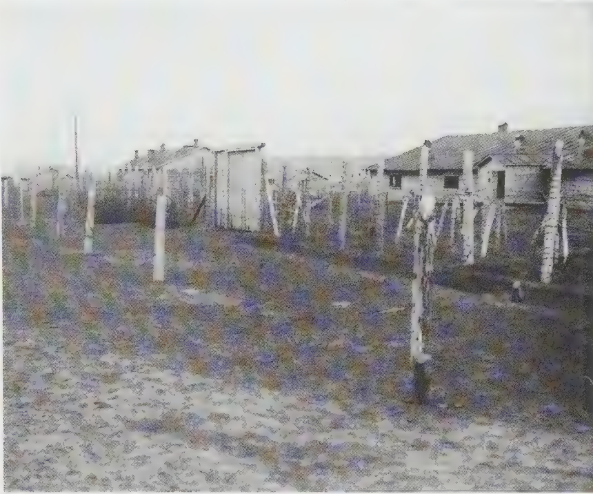
Barracks at a prison camp in the Ural Mountains, 1919–1920. The high rates of illness and death among prisoners testify to the harsh living and working conditions in the Gulag.
