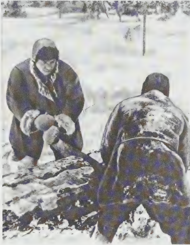
The construction of the Belomor Canal in 1934 required workers to toil in harsh conditions. Here, two prisoners saw wood in knee-deep snow.
